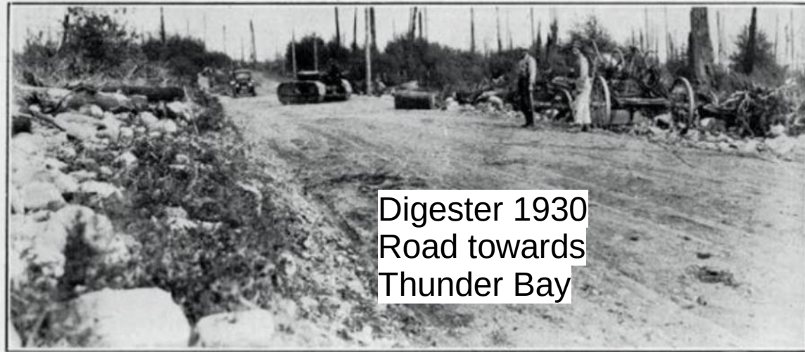
Road work progressing along the Powell River-Thunder Bay Highway. The scene shows the tractor at work widening the road near Lang Bay
